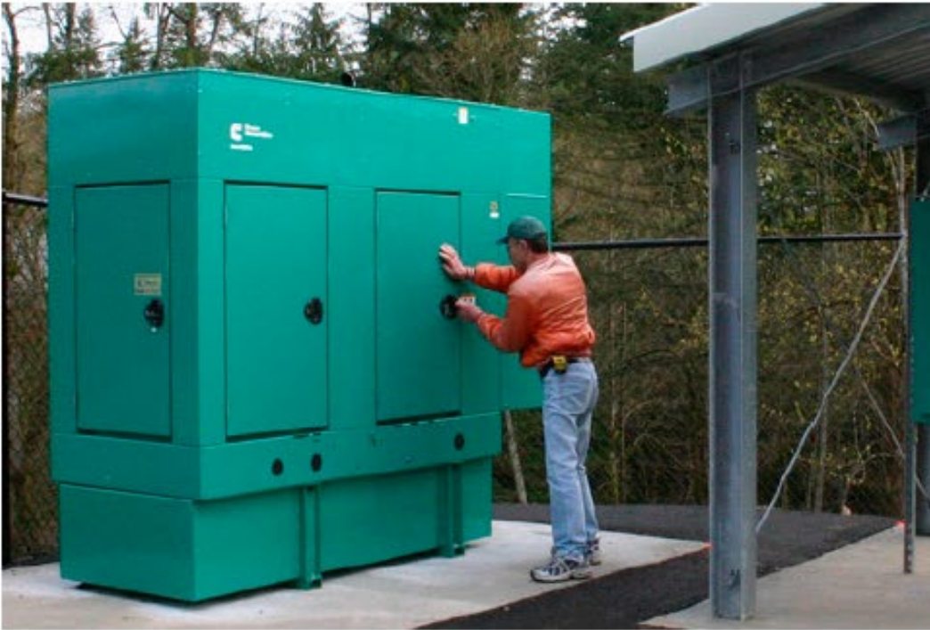
At sites with permanently installed standby generators, factory enclosures provide high security in addition to sound-attenuation.
